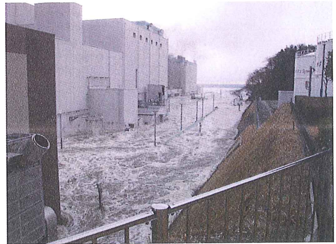
Scenes of the tsunami: Pictures from the neighbouring Fukushima Daiichi plant 10km south showing (a) plant just before tsunami (b) inundated by tsunami. Inundated ground level was 12m above sea level.
